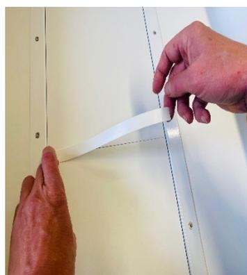
6. Then stick the white adhesive strip over the groove of the two insert plates.
